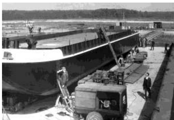
Prace na pochylni
